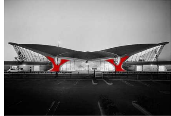
BUTTRESS (COLUMN) SUPPORTS
